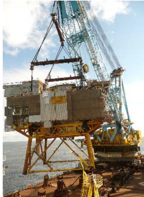
Photograph provided by Total showing Frigg QP topsides lift.
