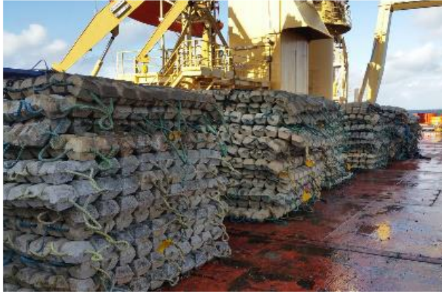
Photograph provided by Fairfield showing concrete mattresses from Dunlin, Merlin & Osprey fields recovered to deck.
