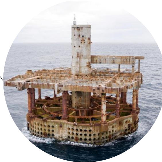
Photograph provided by Total showing Frigg MCP-01 substructure following topsides removal
